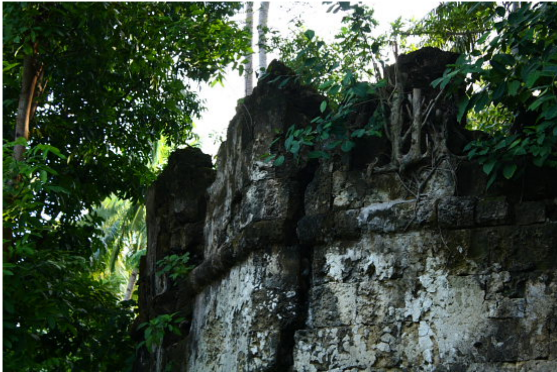
Details of the watchtower's parapet.
