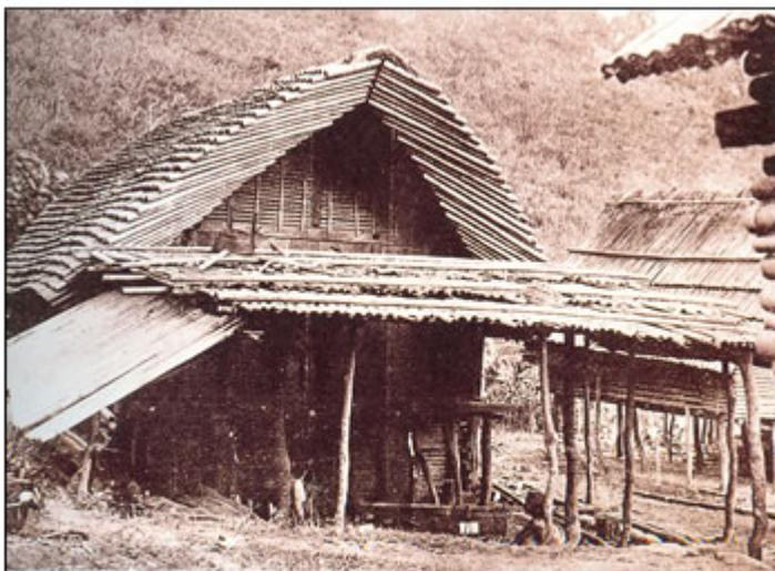
*UPLAND HOMES. The Isneg house binuron, built slightly above the ground, is also a one-room dwelling like the fale but has more light and is bigger. It's bamboo layered, gabled roof ensembles an inverted boat, a design unique to the Isneg who are boatbuilders.*
