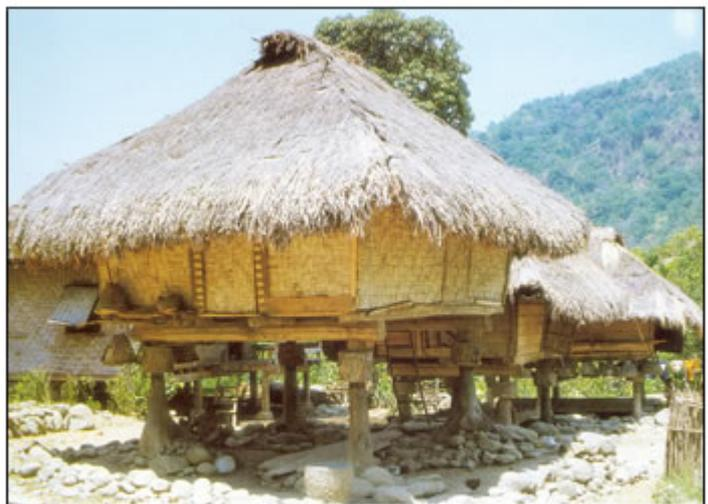
*MOUNTAIN HOUSE. The thick roof of the Ifugao fale and its windowless house cage protect the occupants from the cold, the sun and the rains. The shoulder-high posts, fitted with rat guards below the girders, prevent dampness and vermin from entering the house.*
